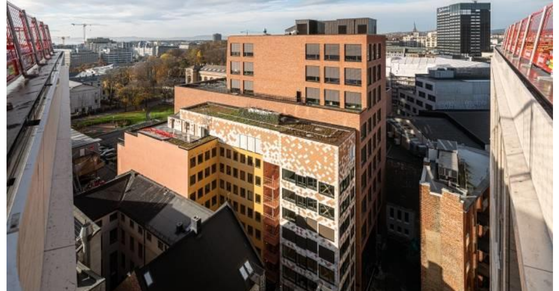
Tulinløkka, rehabilitation 1950's offices
